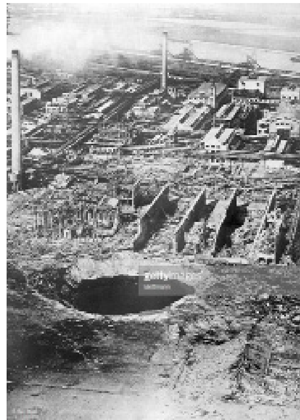
Half the silo that exploded was underground, producing a huge crater, but absorbing much of the potential blast wave. Photo: Getty.
